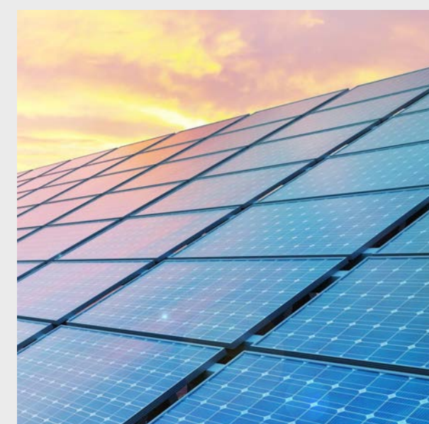
ISL commences 6.4 MW Solar Project at its manufacturing facility in Karachi.
